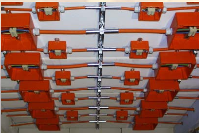
ROSE E30 enclosures comply with all requirements for fire certification in accordance with DIN 4102 part 12
