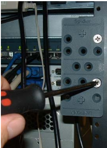
1. Mount the bracket with a Phillips-head screwdriver
