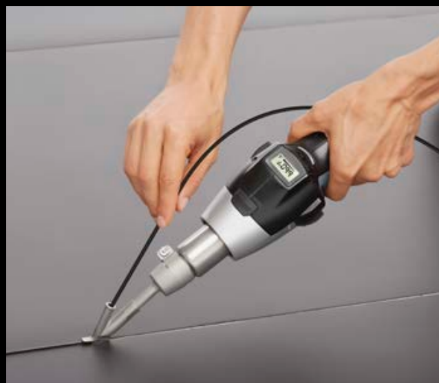
Welding linoleum floors.
