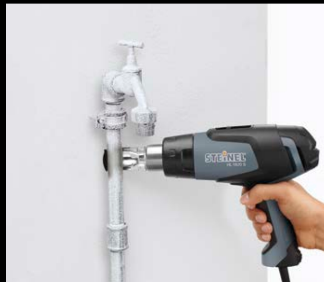
Thawing frozen pipes.
