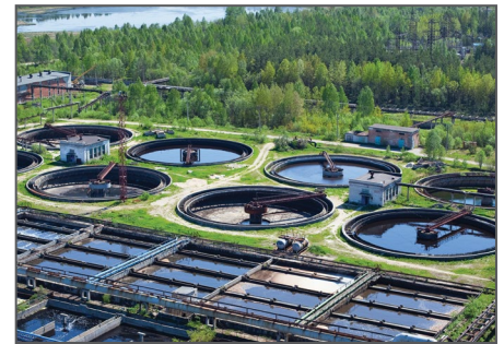
Water, wastewater treatment
