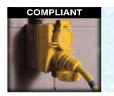
3) Do we have 15 or 20 amp, 125 or 250 volt receptacles installed in wet locations that are NOT weatherproof with or without the attachment plug inserted?
