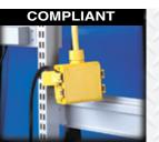
4) Are pendant applications (flexible cord drop from the ceiling without structural support) using boxes that are NOT listed for pendant applications?
