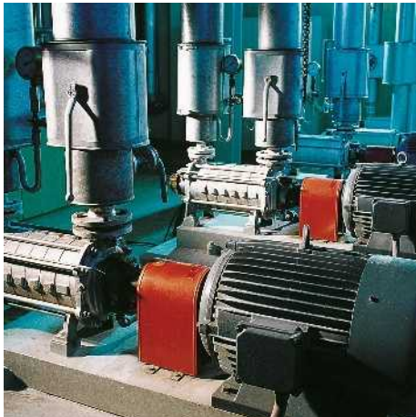
Protection against dry running, blocking, and cavitation, warning thresholds to indicate filter contamination.
