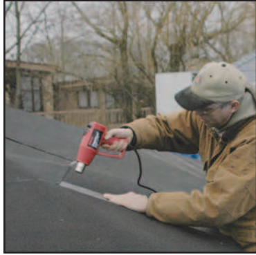
Weld Roofing Membrane
