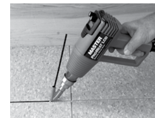
Welding Flooring Material
