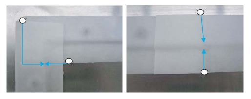
In the above images, the white circles indicate where 3M 4000UV should be applied in the corner and step situations. These two general categories can describe most common configurations. For configurations other than these, the general principle is to use 3M<sup>TM</sup> 4000UV in any place where water (shown as blue arrows) could seep past an improperly joined overlap.
