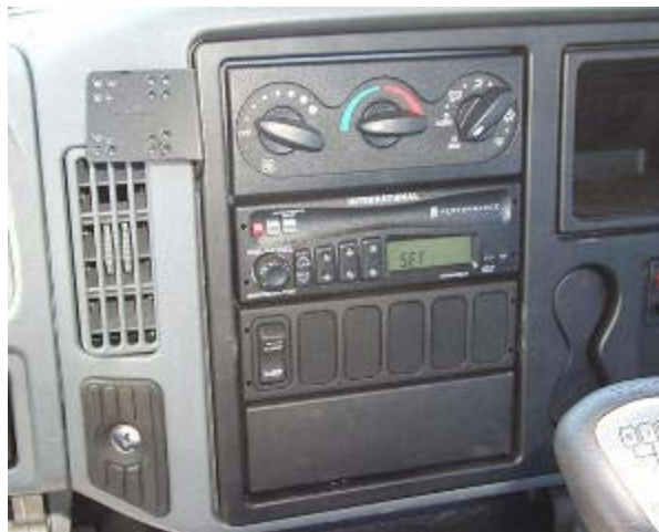
Prototype installed showing location Finished Install Picture
