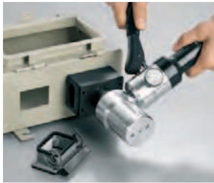
Automatic centre punching at the drill points when punching out holes for heavy-duty connectors.
