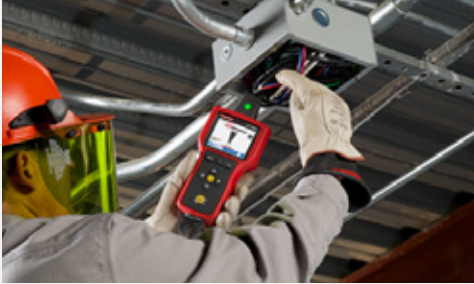
Trace energized or de-energized wires by removing the junction box cover.
