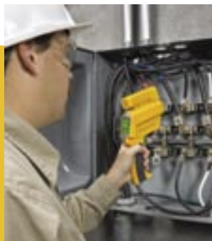
1 Log temperature and take photo with the Fluke 576.
