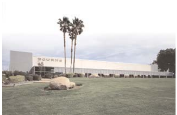
Bourns Corporate headquarters in Riverside, California
