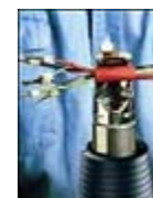
Applying Shrink Tubes
