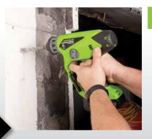
Air-Coupling Hammer Mechanism provides quick hole drilling in hard concrete!
