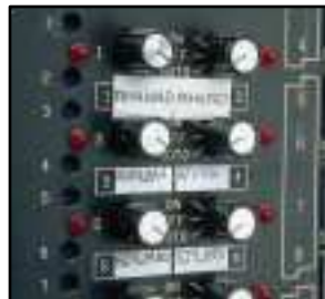
Label switches, relays and other devices
