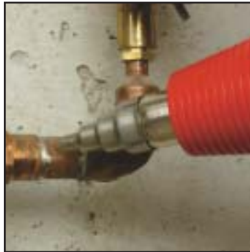
Solder Copper Pipe
