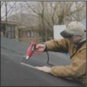
Weld Roofing Felt
