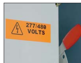
Safety & Facility ID
