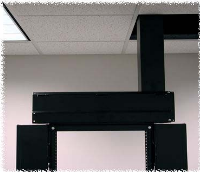
DNRR_HD Relay Rack with: Installed top manager (Double). With left & right vertical mangers. Chimney through ceiling.
