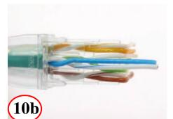
Check Blu pair for alignment Add ½ twist if necessary
