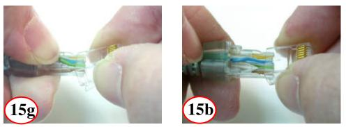
Place load bar assembly into housing
