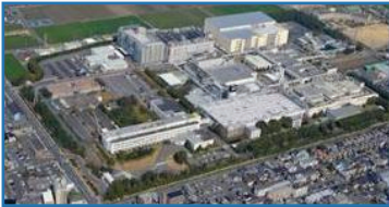
Shiga: Kyocera Display Corp HQ & Yasu Plant (JAPAN)
