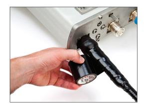
3.5 Starting 1" (25 mm) below the previous layer of vinyl tape, wrap the entire cable and connection section with three continuous half-lapped layers of ¾" (19 mm) wide vinyl tape.
