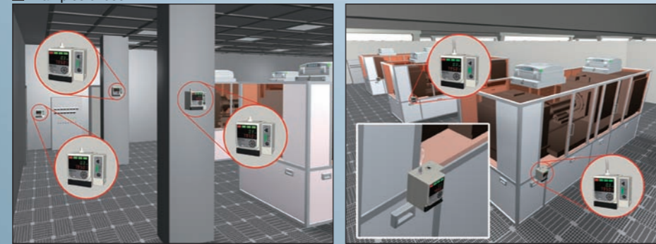
Multi-point continuous monitoring in clean room
